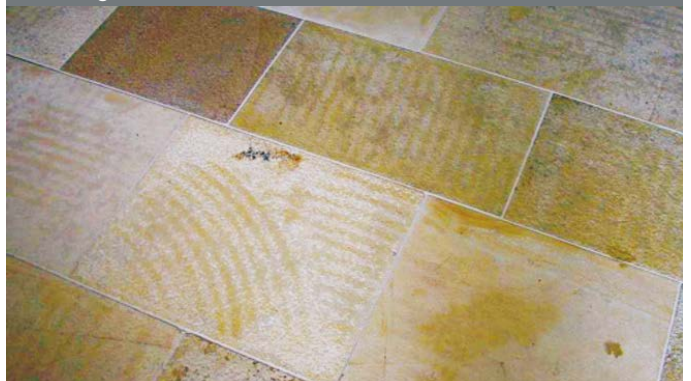
Staining in natural stone and reconstituted stone
