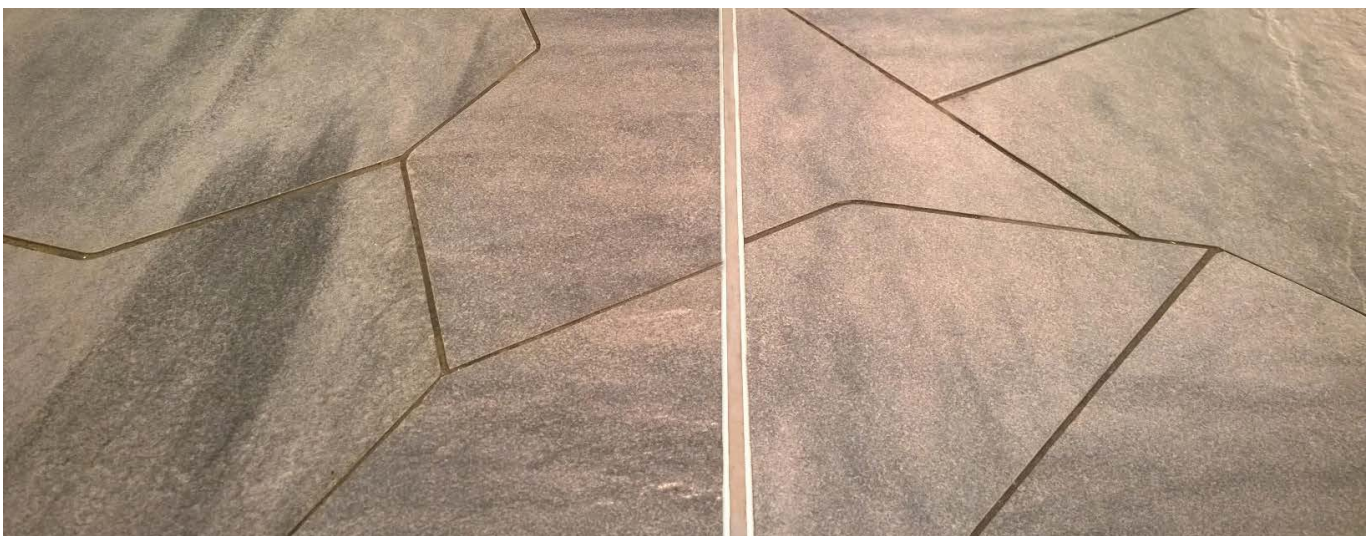
Movement joint protected by metal divider strips and filled with MasterSeal® trafficable elastomeric joint sealants.
